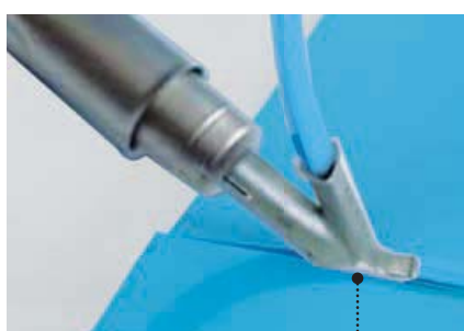
Welding by means of electrodes for mobile use
